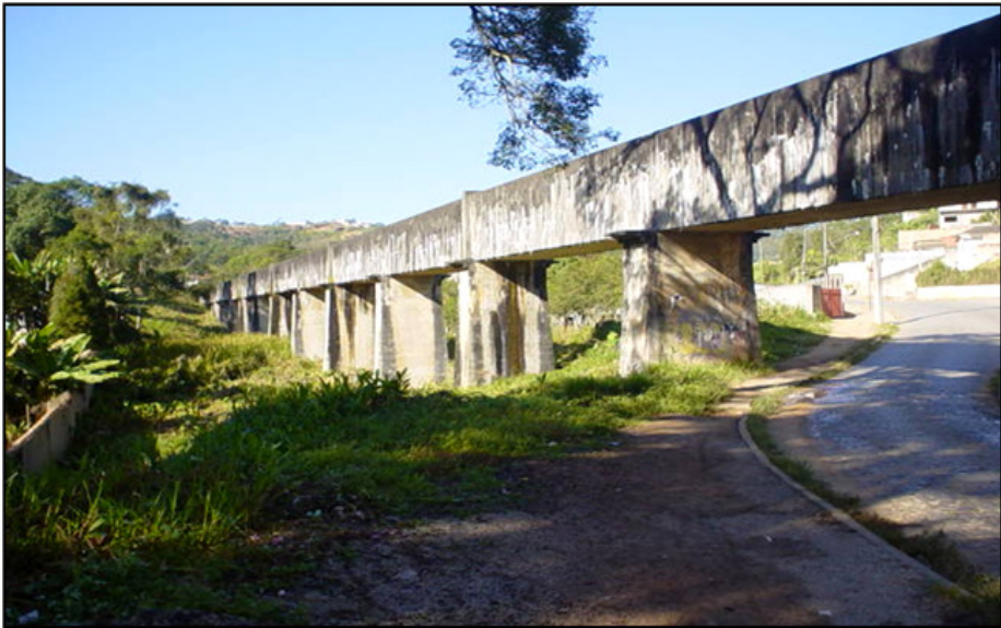
Figure 6 - Rio Claro system aqueduct
